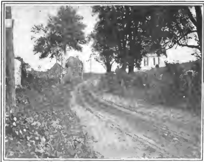
Winding country road near Greenville—this is full of small bumps
